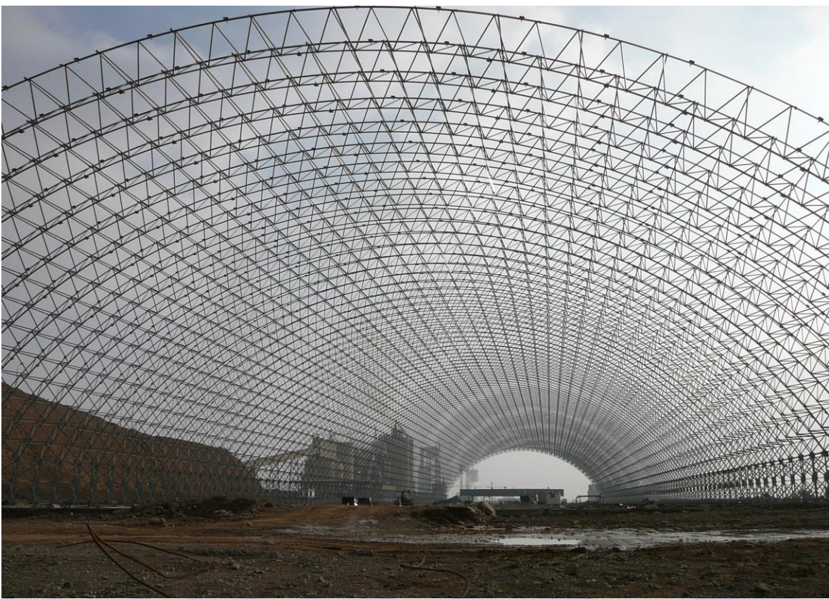
Red Soil and Lime Stone shelters of Soofian cement project
